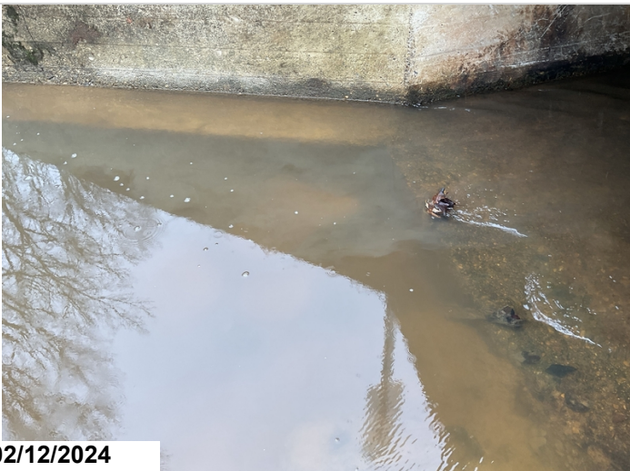
Scour to footing at inlet end.
