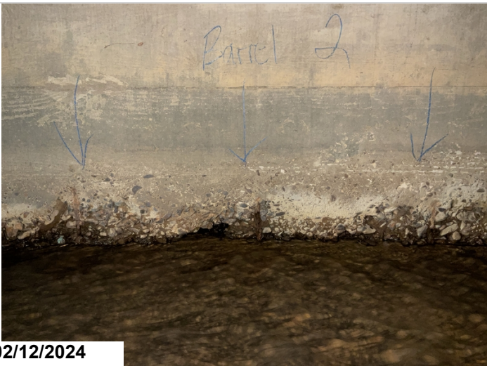
Barrel 2 abrasion with rebar exposed. CS3
