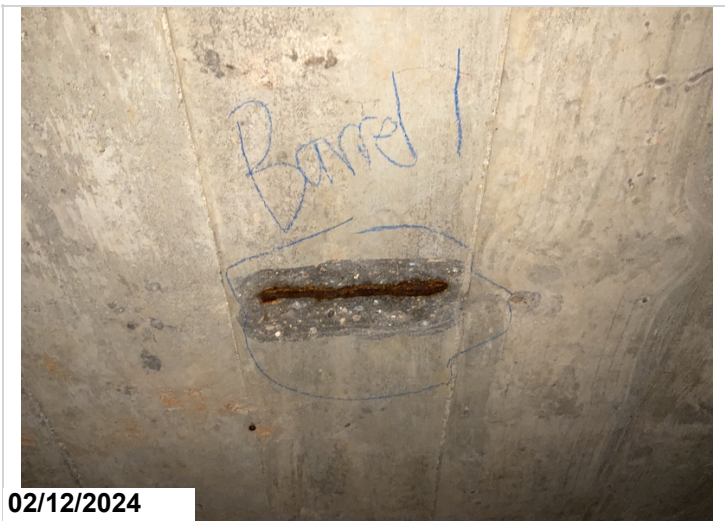
Exposed rebar in barrel 1. CS3
