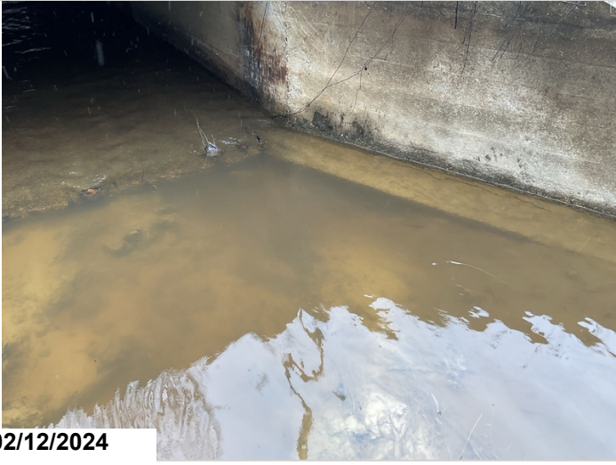
Scour to footing at inlet end.
