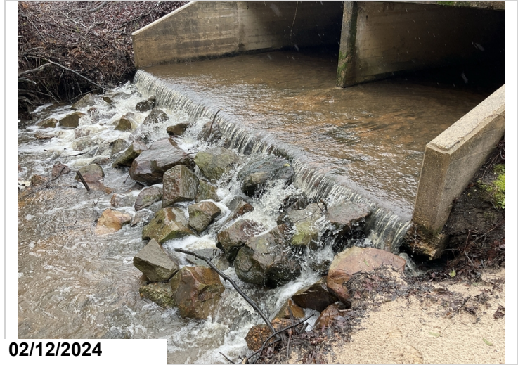
Repairs from past scour
