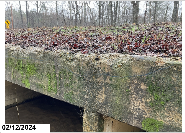
Spalling on outlet end headwall. CS2
