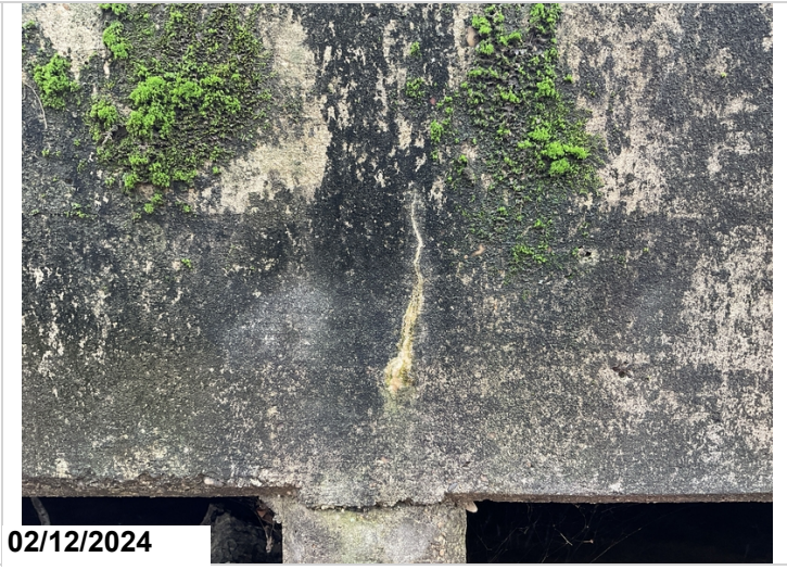
Efflorescence to inlet end headwall. CS2
