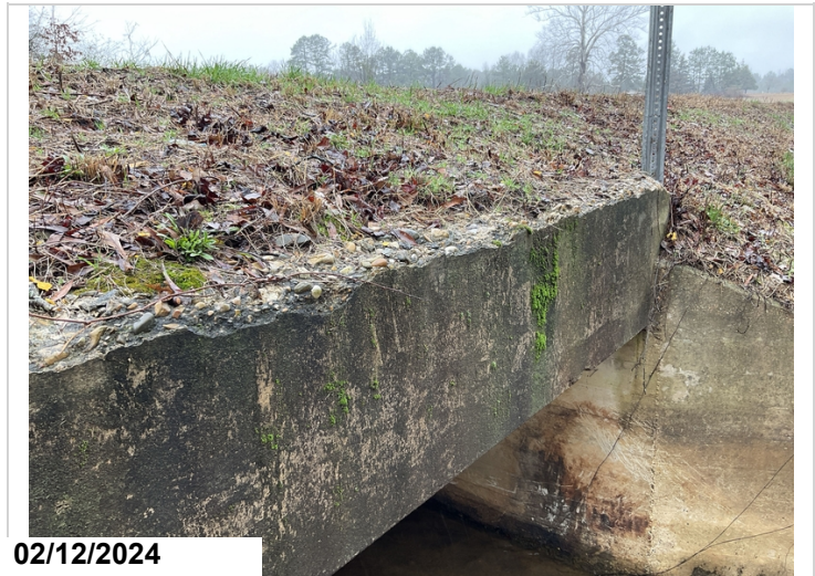
Spalling to inlet end headwall above barrel 1. CS2
