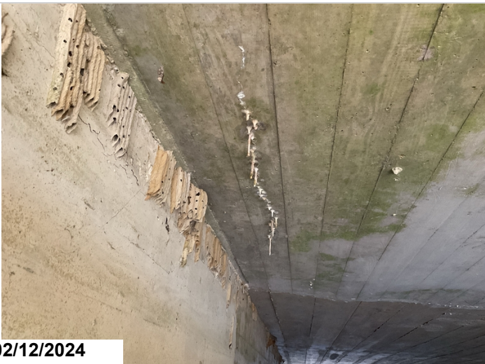
Barrel 1 cracking with efflorescence. CS2
