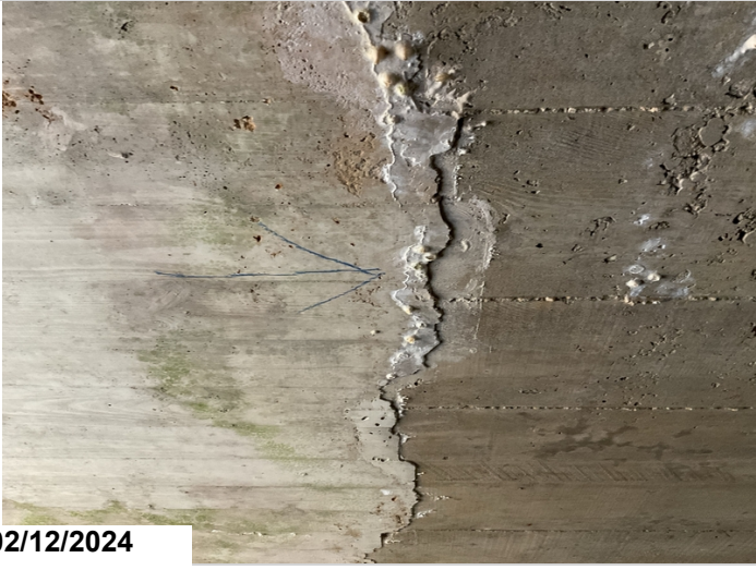
Barrel 1 cracking with efflorescence. CS2
