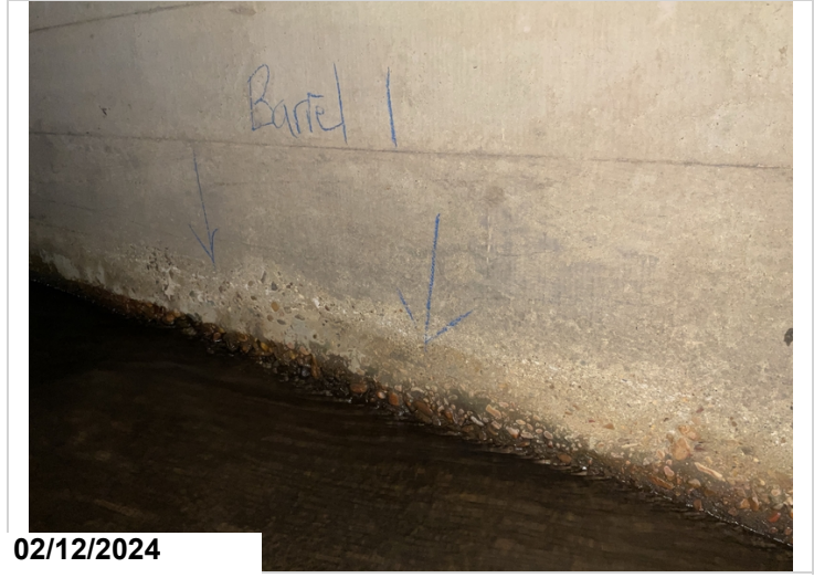
Barrel 1 abrasion. CS3
