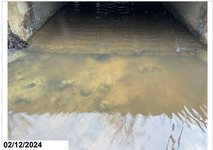
Scour to footing at inlet end.
