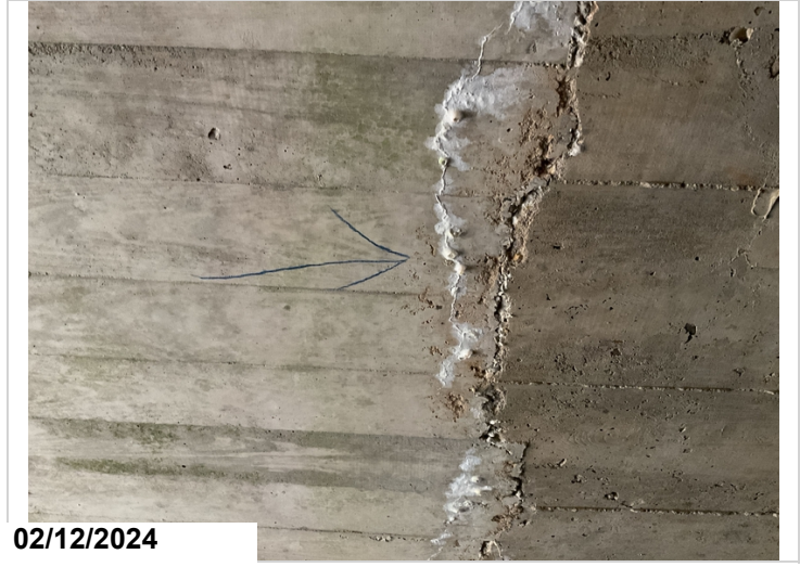
Barrel 2 cracking with efflorescence. CS2
