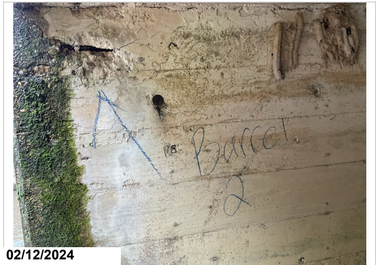
Barrel 2 rebar exposed at outlet end near divider wall. CS3
