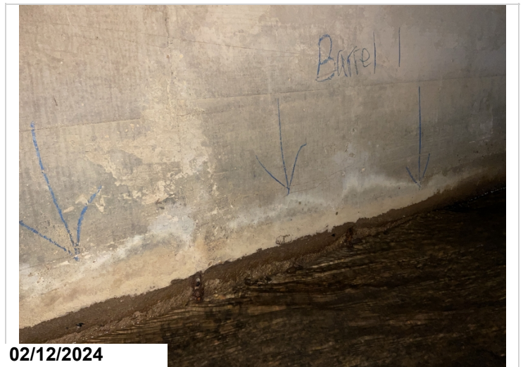
Barrel 1 abrasion. CS3
